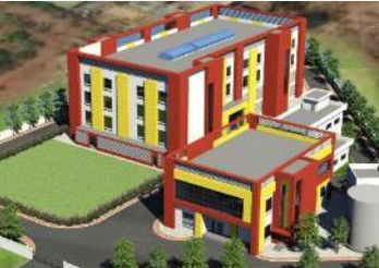
Additional Manufacturing Facility (200 KL), Bidar
